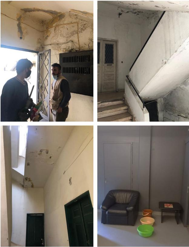
**Figure 6:** The images above were taken from inside the residential buildings, showing traces of severe mold, humidity, and dampness. Source: Abir Cheaitli, 2021.
