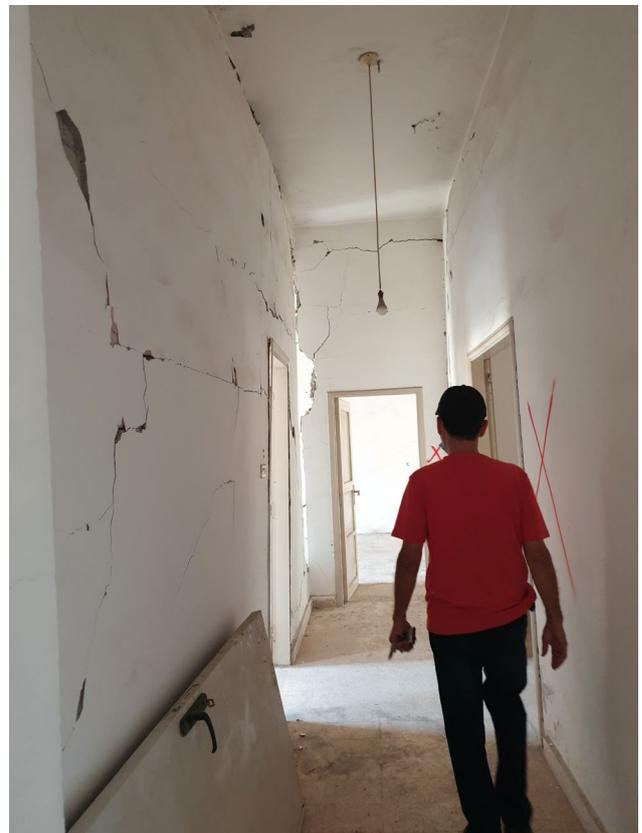
**Figure 38.** A structurally damaged residential apartment in AL-Khodor sub-neighborhood by the port blast.
