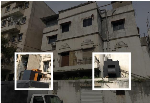
**Figure 29c.** Two private generators that are located at the top floor of a building because of the lack of space on the ground level. Source: Abir Cheaitli, 2021.
