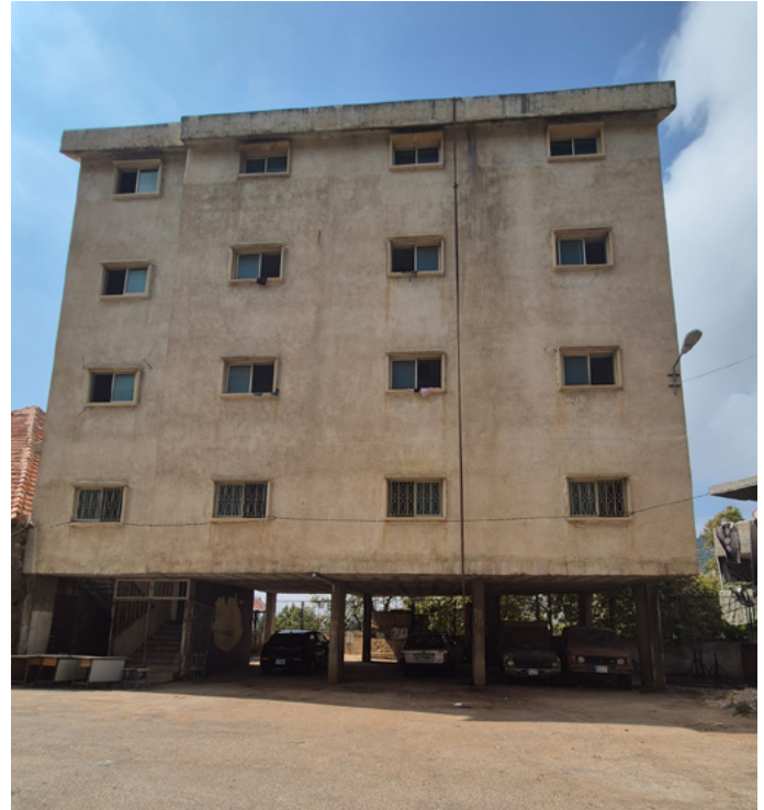
Figure 10. OCA designated shelter building in Baskinta (own photo)
