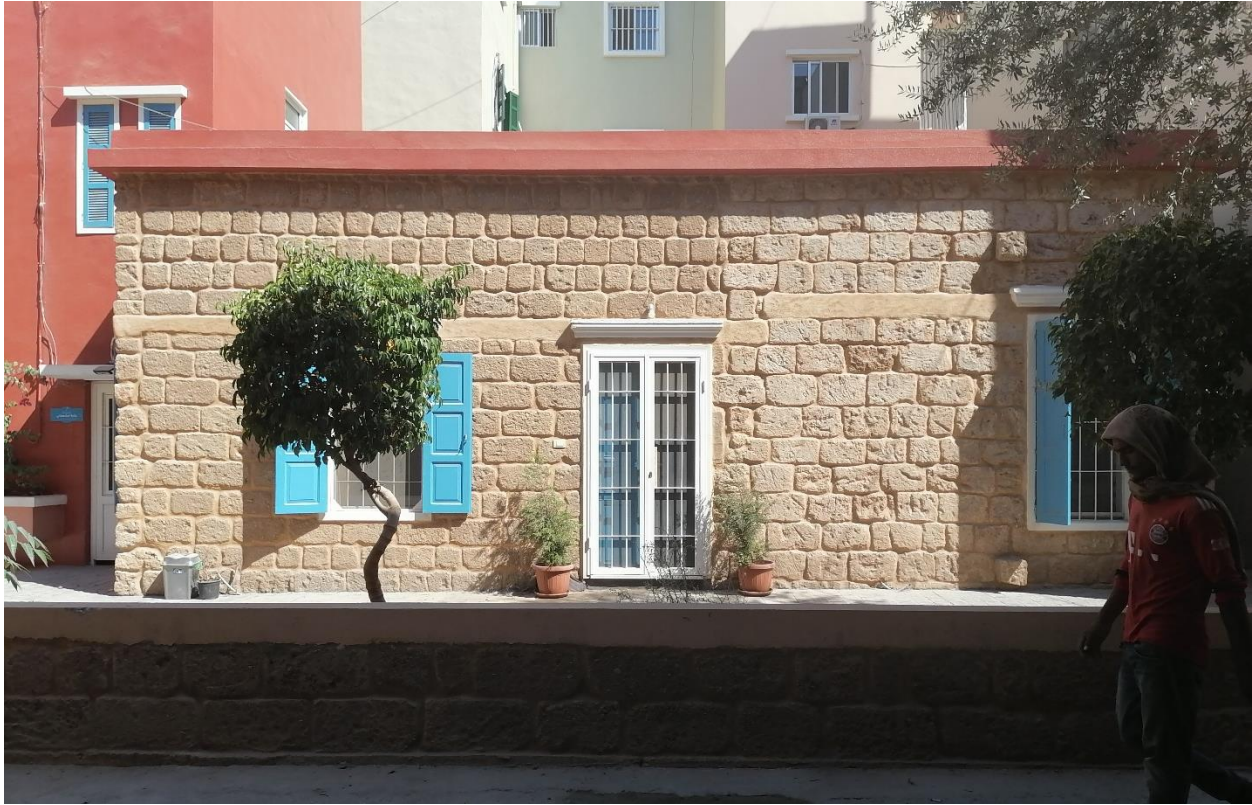
Figure 33: Neighborhood scale repair undertaken by one NGO. September 2021. Photo: Abir Zaatari.
