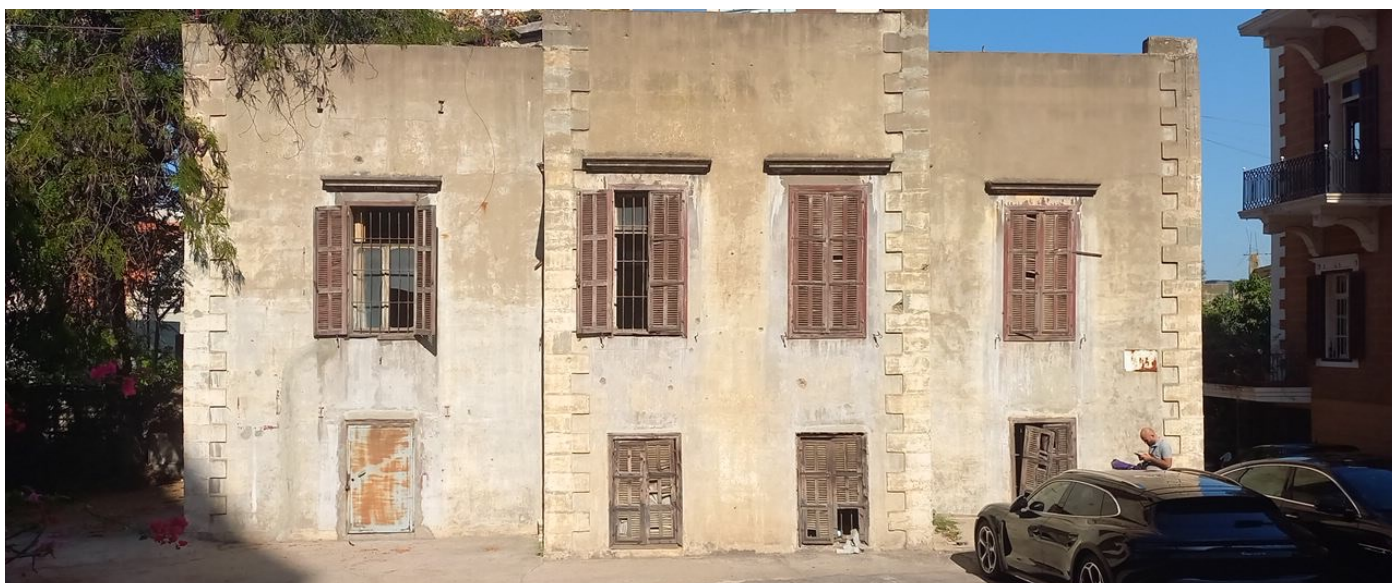
Figure 1. A Vacant Building in Beirut, Source: Beirut Urban Lab Vacancy Survey, 2023
