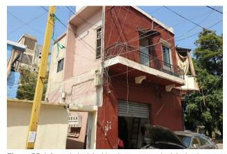
**Figure 39.** Informal electrical hook-ups on an electrical pole. Source: Batoul Yassine, 2021.
