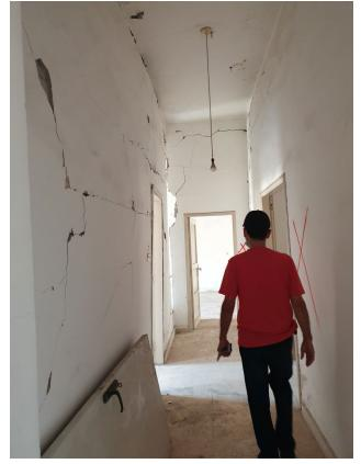
**Figure 38.** A structurally damaged residential apartment in AL-Khodor sub-neighborhood by the port blast. Source: Batoul Yassine, 2021.
