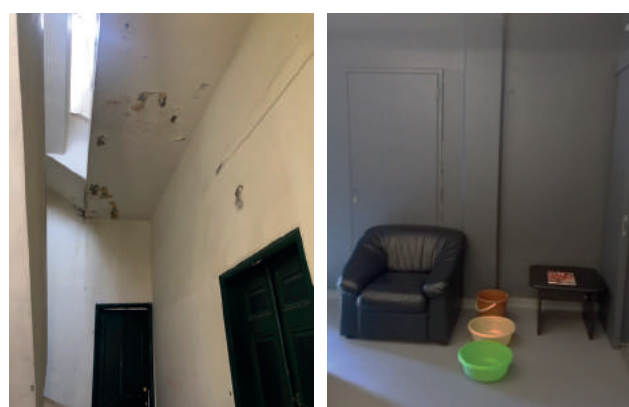
Figure 6: The images above were taken from inside the residential buildings, showing traces of severe mold, humidity, and dampness. Source: Abir Cheaitli, 2021.
