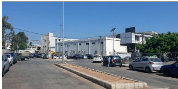
Figure 28. Karantina’s government hospital. Source: Abir Cheaitli, 2021.
