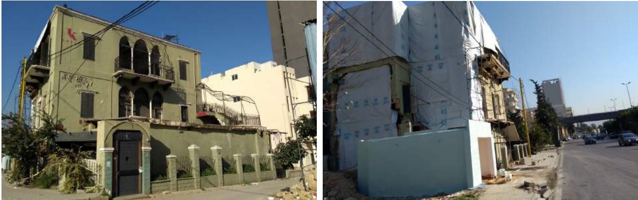
Figure 71 and 72. Harbor 201 after the port blast. Source: Ali Ghaddar, 2021.
