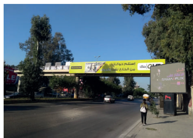
Figure 6. A pedestrian overpass that links Karantina to Mar Mikhael. Source: Ali Ghaddar, 2021.
