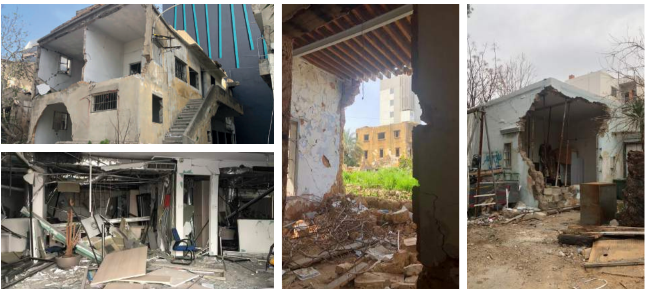
Figure 8: Collapsed buildings after the port blast in Karantina. Source: Abir Cheaitli, 2021.
