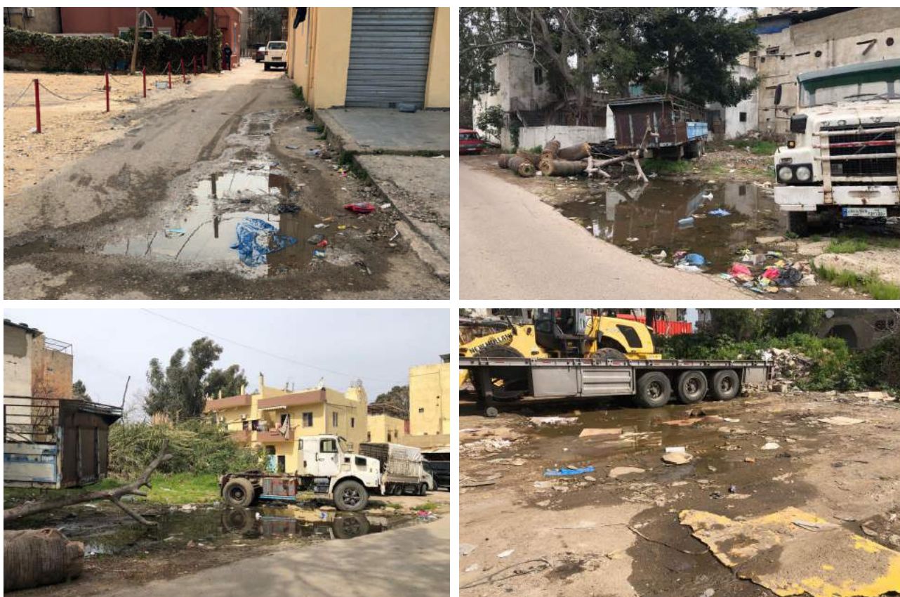
Figure 33. Wastewater discharged on streets and vacant lots. Source: Abir Cheaitli, 2021.
