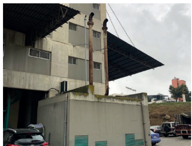
Figure 29a: The electrical generator of the Bakalian flourmills. Source: Abir Cheaitli, 2021.
