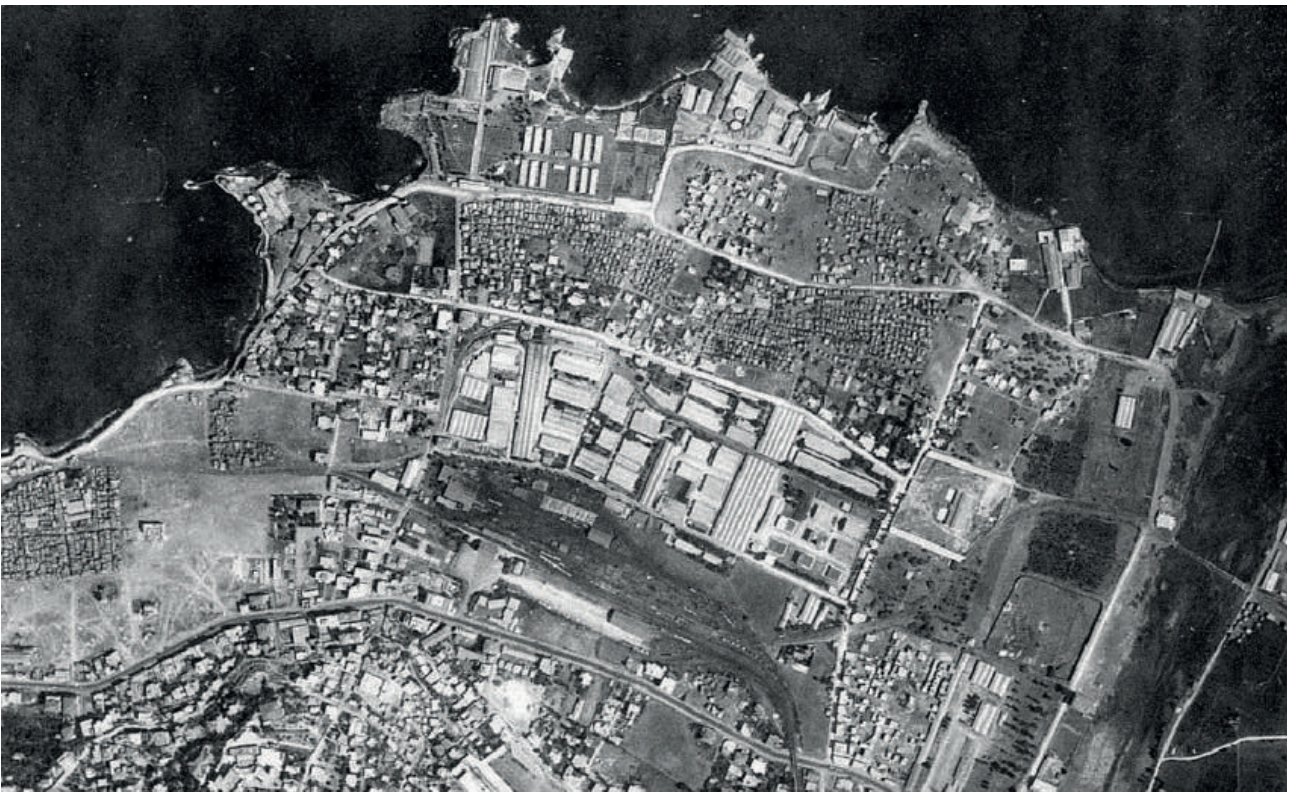
Figure 7: Aerial Photo, taken in 1931, showing Armenian and refugee Tanke settlements. Source: Sandra Frem, 2009.
