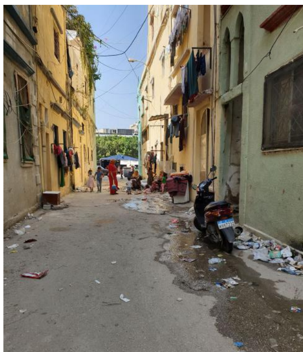
Figure 23. An alleyway in Al-Khodor sub-neighborhood. Source: Batoul Yassine, 2020.
