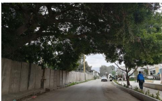
Figure 19. Military concrete fenced walls in Al-Khodor sub-neighborhood. Source: Abir Cheaitli, 2021.
