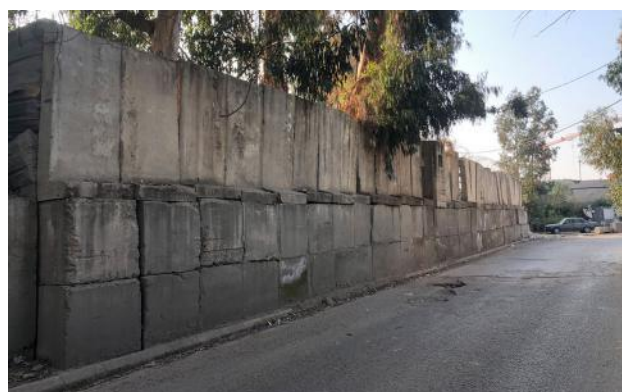
Figure 20. Other military concrete fenced walls in the industrial area. Source: Abir Cheaitli, 2021.
