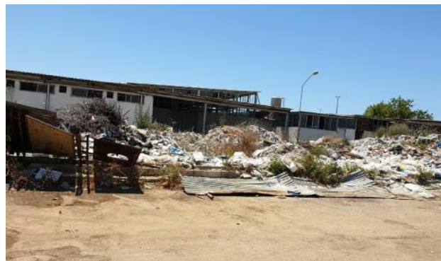
Figure 5. The dilapidated condition of the current slaughterhouse in Karantina. Source: Abir Cheaitli , 2021.
