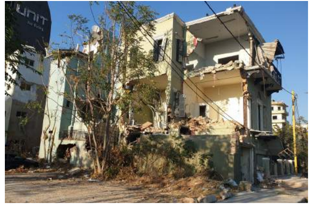
Figure 3. A damaged building in Karantina. Source: Batoul Yassine, 2020.
