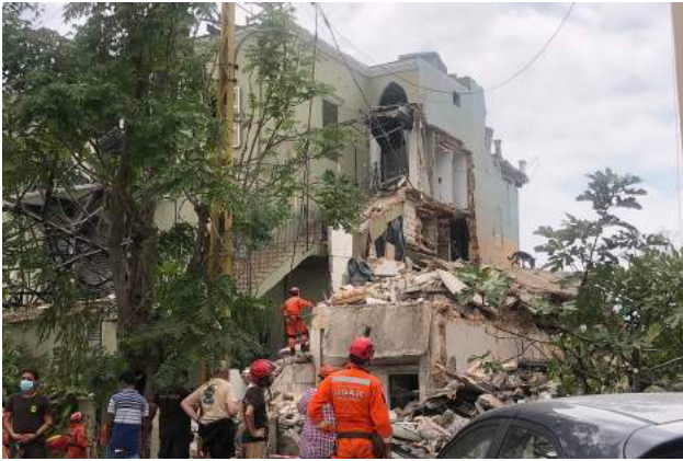
Figure 2. Rescue efforts in a collapsed building in Karantina. Source: Hayfaa Abou Ibrahim, 2020.
