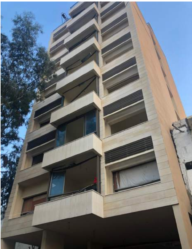
Figure 12. New buildings constructed in Karantina. Source: Abir Cheaitli, 2020.
