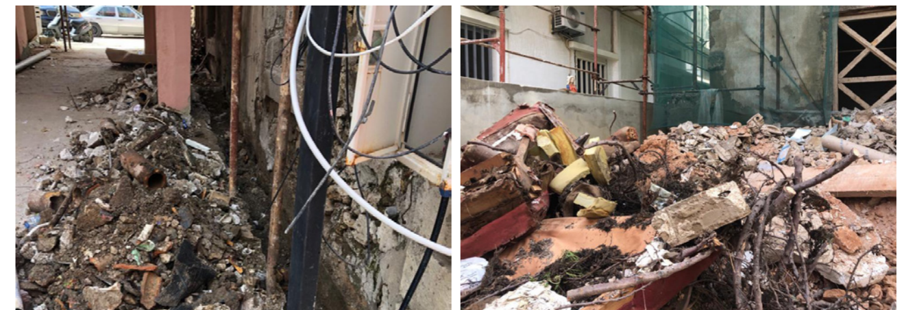
Figure 40. Construction and demolition waste from the port blast. Source: Abir Cheaitli, 2021.
