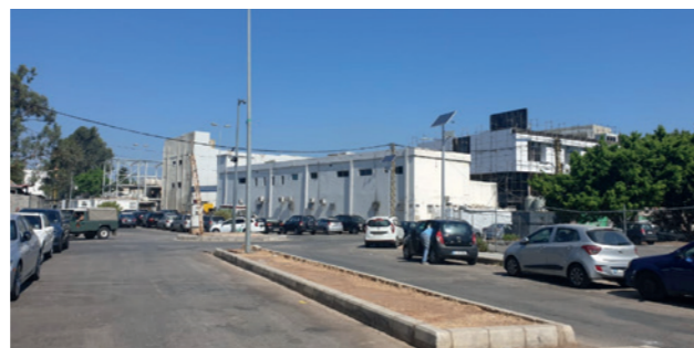
Figure 28. Karantina’s government hospital. Source: Abir Cheaitli, 2021.
