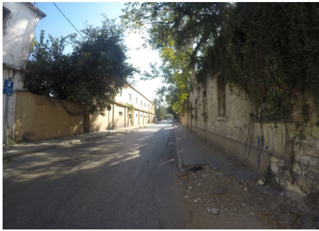
Figure 35. The degraded quality of the sidewalks in Karantina. Source: Abir Cheaitli, 2021.
