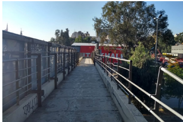
Figure 7. The physical quality of the pedestrian overpass from Karantina to Mar Mikhael: the structure of the overpass does not include a shaded roof and the handrail is damaged. Source: Ali Ghaddar, 2021.
