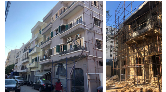
Figure 9. Two distinct building typologies. Source: Abir Cheaitli, 2020.
