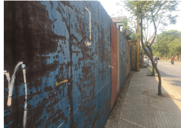
Figure 16. The inaccessible wall of the municipal lot from Al-Rehban Street. Source: Abir Cheaitli, 2021.
