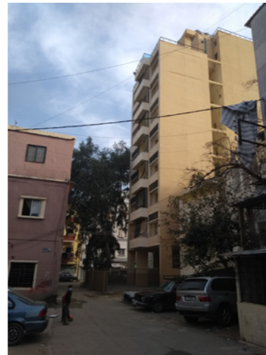
Figure 7. A newly constructed building in Al-Khodor sub-neighborhood. Source: Abir Cheaitli, 2021.
