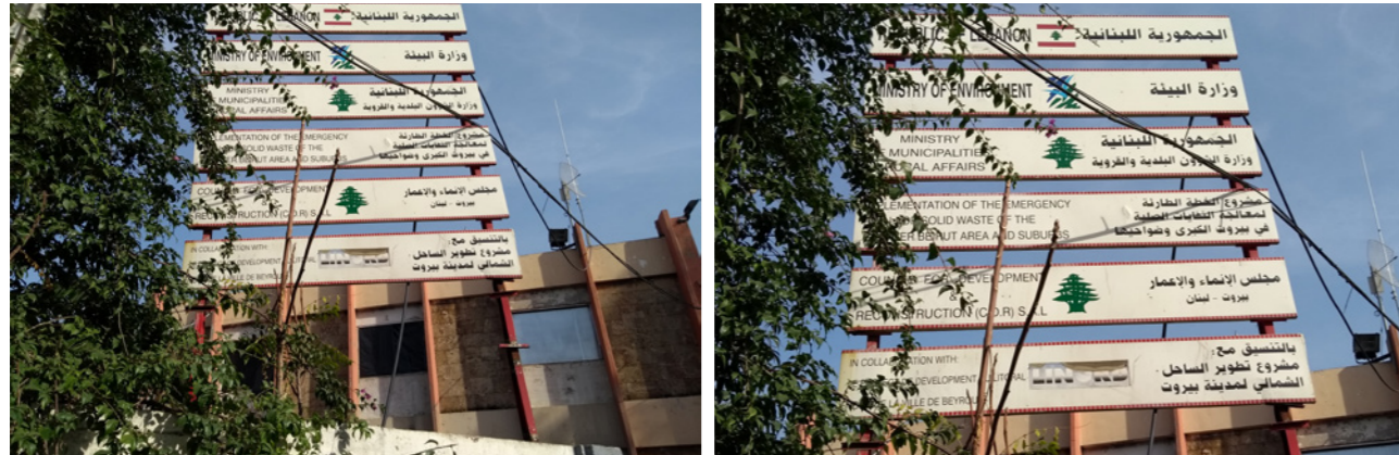
Figure 34. The panel at the entrance of the solid waste management facility mentions the collaboration with the LINORD Project. Source: Ali Ghaddar, 2021.
