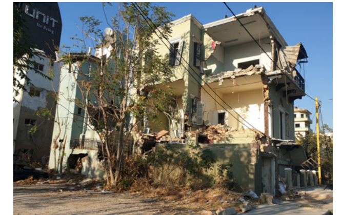
Figure 3. A damaged building in Karantina. Source: Batoul Yassine, 2020.
