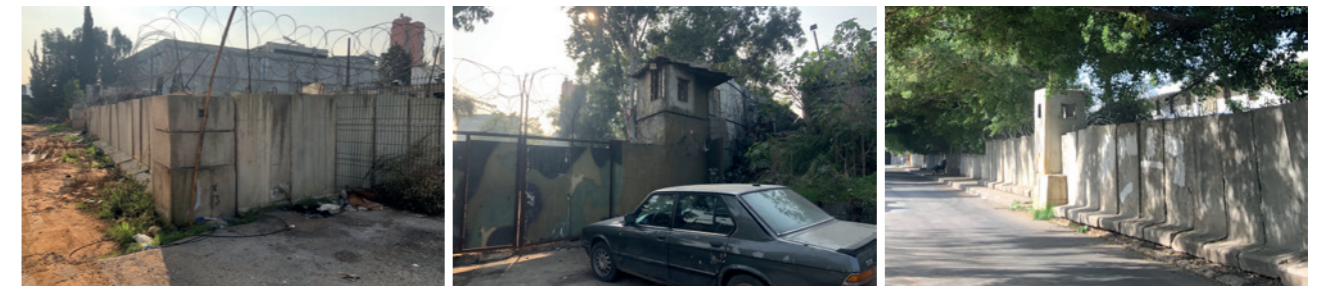
Figure 25. Edge conditions and security elements along the militarized lots. Source: Abir Cheaitli, 2021.
