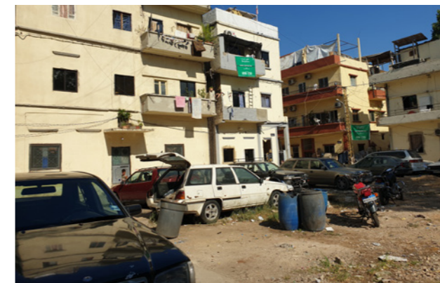
Figure 1. Residential buildings in Al-Khodor sub-neighborhood Source: Batoul Yassine, 2021.
