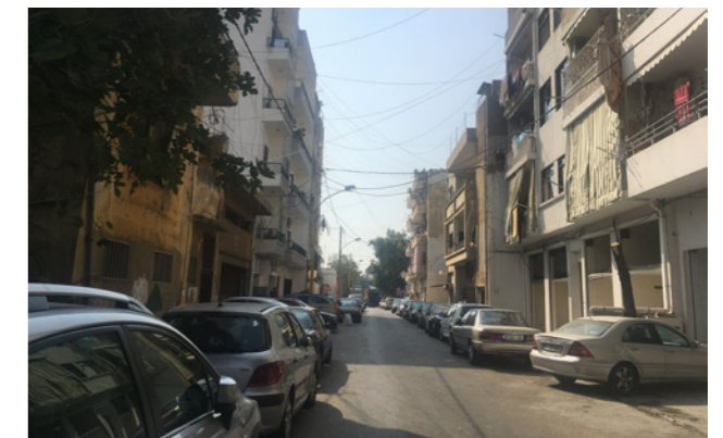
Figure 2. Residential buildings in Al-Senegal sub-neighborhood Source: Rami Shayya, 2022.
